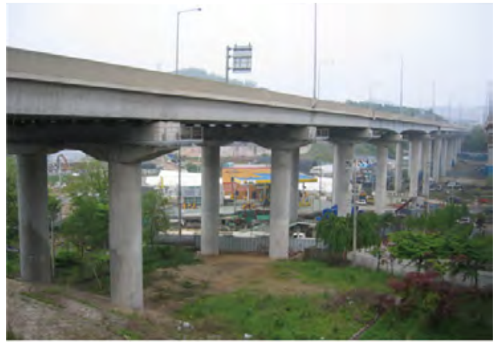
Precision Safety Diagnosis on Sorae Tunnel and 5 others
