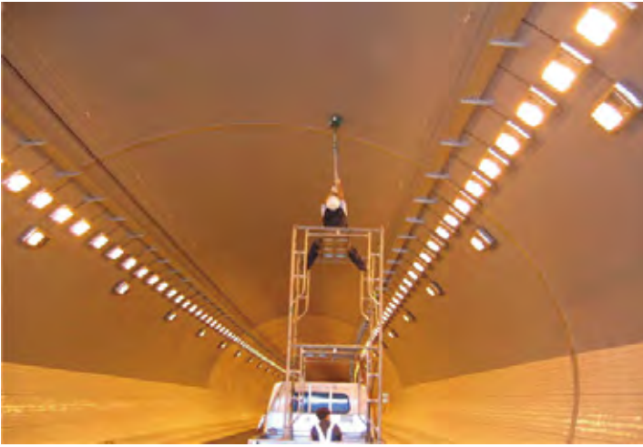
Measurement, Safety Check and Reinforcement Design for Gokdu Tunnel
