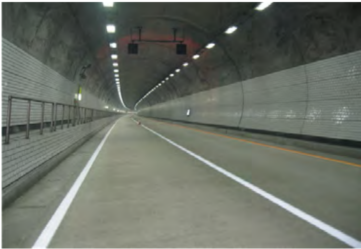
Precision Safety Diagnosis on Geryong Tunnel and 12 others
